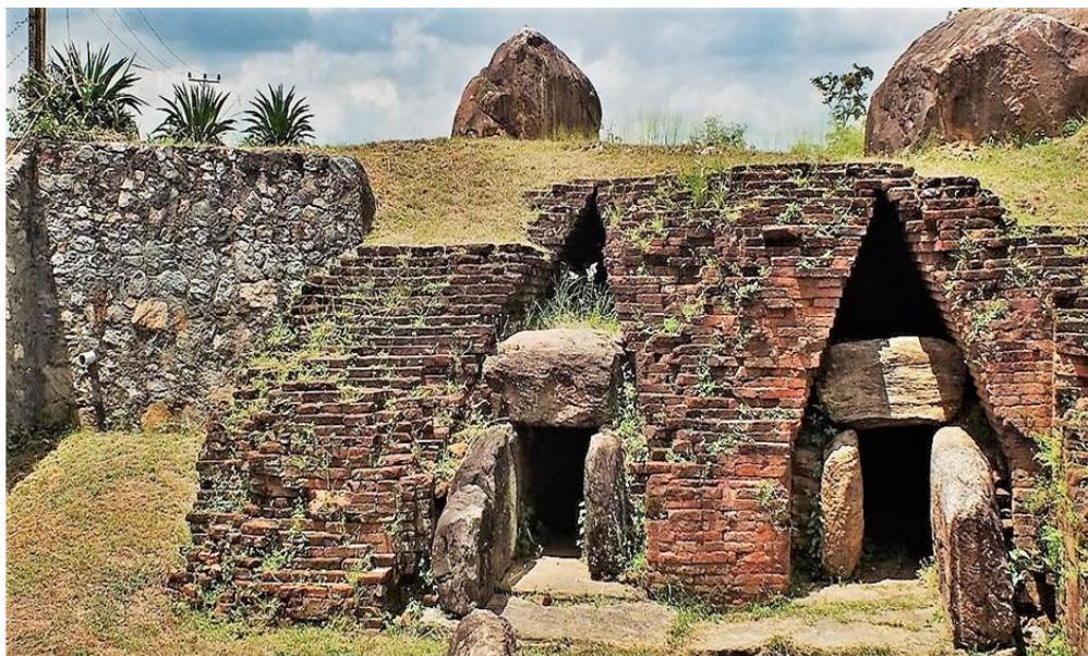
Fig. 2. A photograph of sluice gate (Sorowwa) of the dam of the tank fed by Maduru Oya believed to be built in 4th millennium BC
