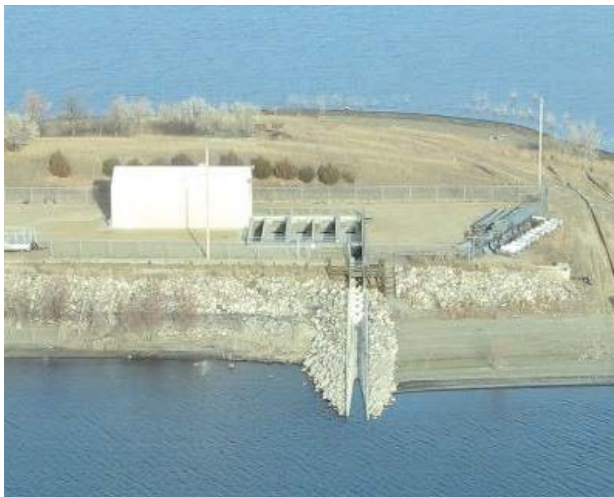
Figure 1. Whitlock Spawning Station on Lake Oahe, South Dakota, USA. Note the building, catch raceways, and fish ladder (this image was taken when the station was not in operation, so no water is in the raceways or ladder).
