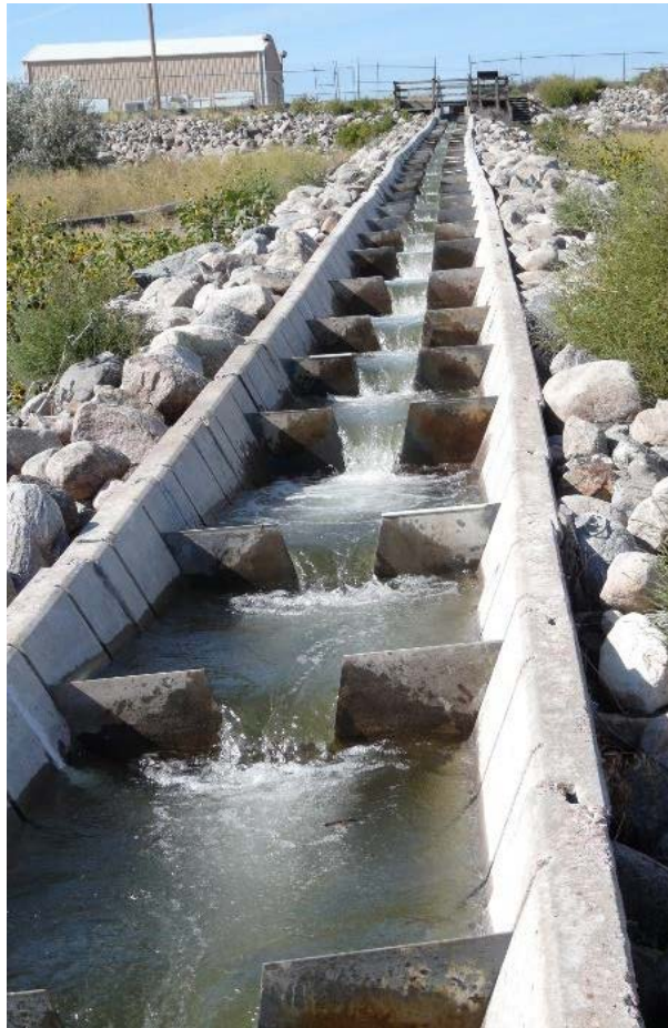
Figure 2. The fish ladder in operation at Whitlock Spawning Station on Lake Oahe, South Dakota, USA.
