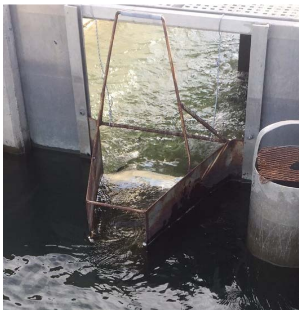
Figure 3. The open weir at the top of the fish ladder at Whitlock Spawning Station on Lake Oahe, South Dakota, USA.
