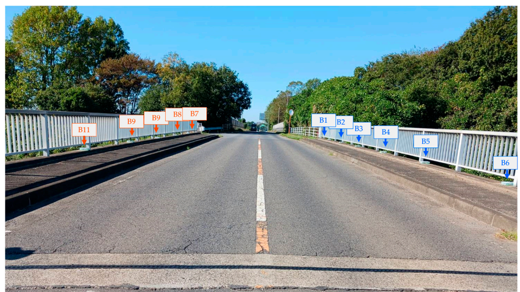
Figure 11. The monitored bridge.
